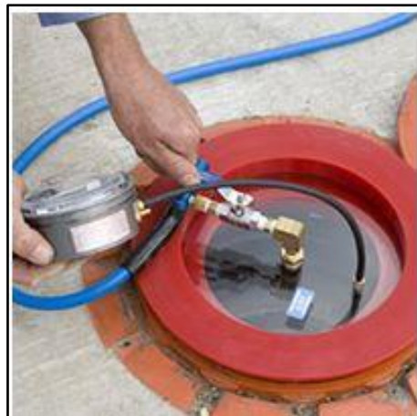
Fig. 13 - Vacuum tightness test on a spill bucket
