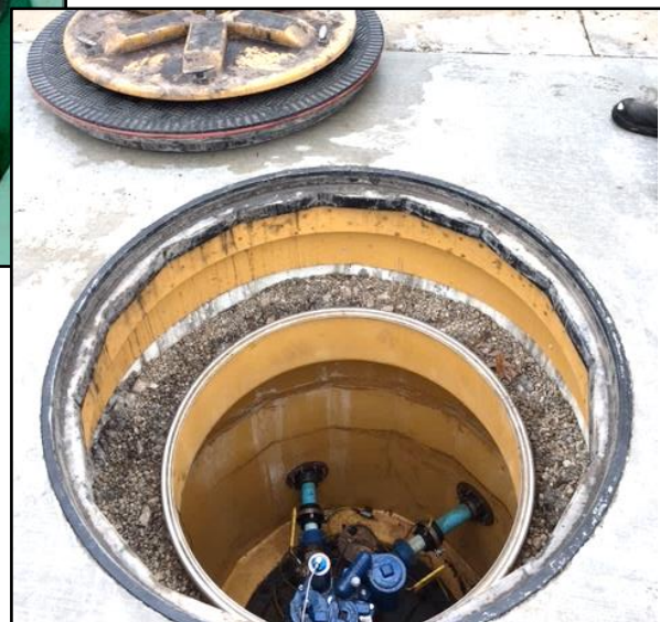
Fig. 10 -top tank containment (TTC) sump at an active facility
