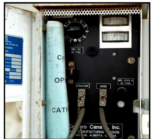
Fig. 17 – Impressed current panel
