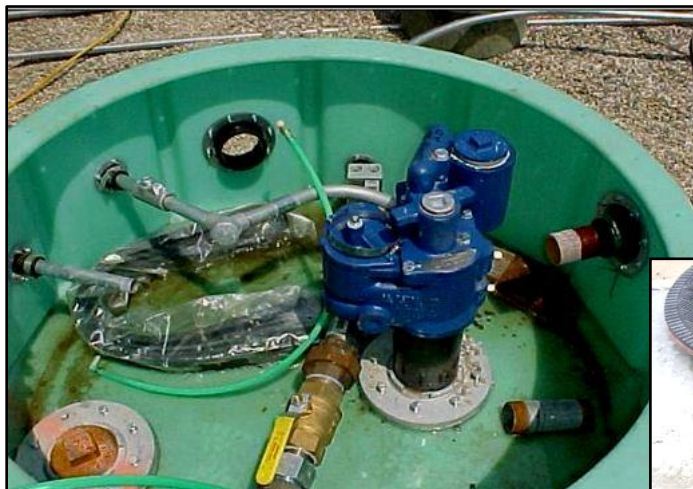
Fig. 9 -top tank containment (TTC) sump undergoing new construction
