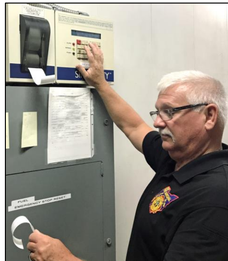
Fig. 4 - Automatic tank gauging (ATG)
