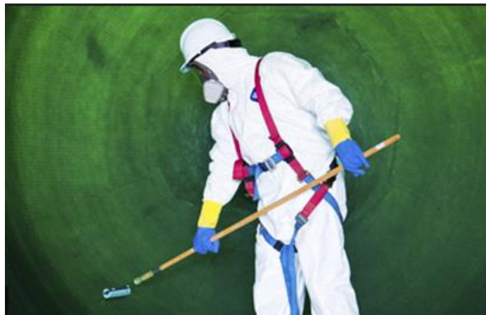
Fig. 20 – Lining of UST
