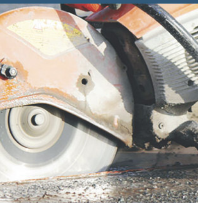
CUTTING NEW CONCRETE
