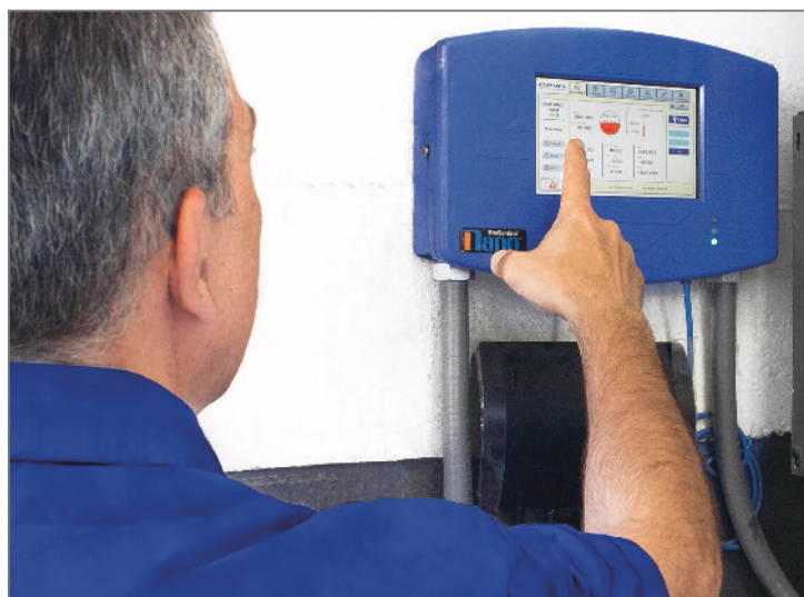
Modern tank gauges, such as OPW's SiteSentinel® Nano® Console shown here, offer an intuitive touchscreen and user-friendly monitoring tools.
